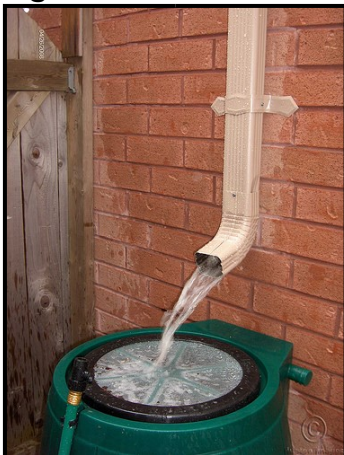
Figure. 4 Rainwater collection (through downpipes and sieves)
