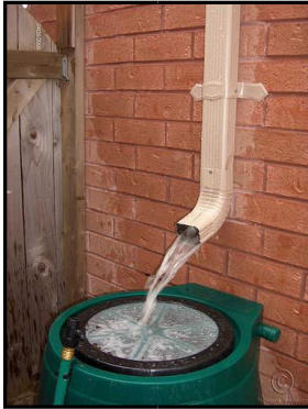
Figure. 4 Rainwater collection (through downpipes and sieves)
